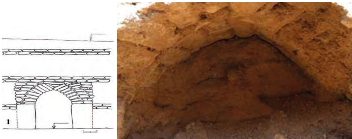
Pic. 5. 1 – reconstruction of the arched block in the northern wall of the room A (passage from the house A in the room B); 2 – loose filling of the top of the same arches. 2012
