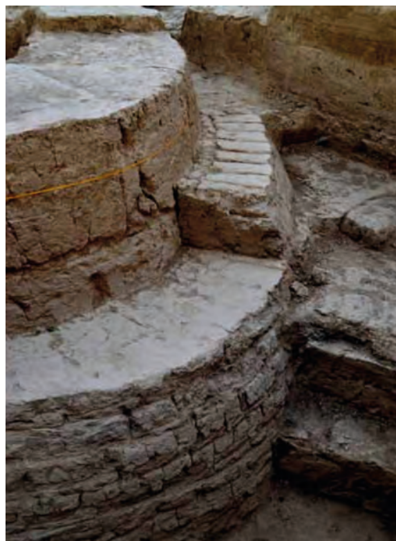
Pic. 8. Laying of walls in CP1 and external lining of walls in CP2
